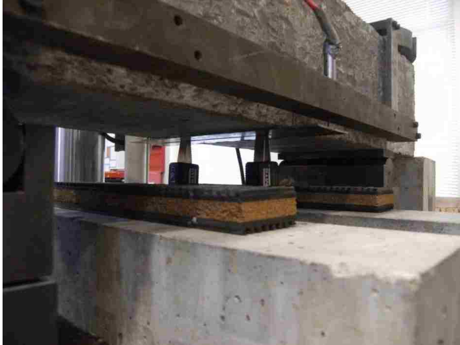
Figure 3.16 – Installation of clip gages
